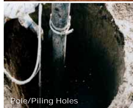
Debris Removal Cleanouts
