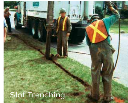
Daylighting/Potholing
