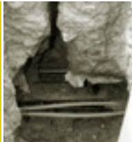
DAYLIGHTING POTHOLING
